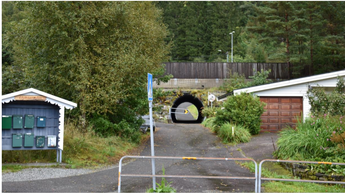
Figur 12: Undergang under E16.
